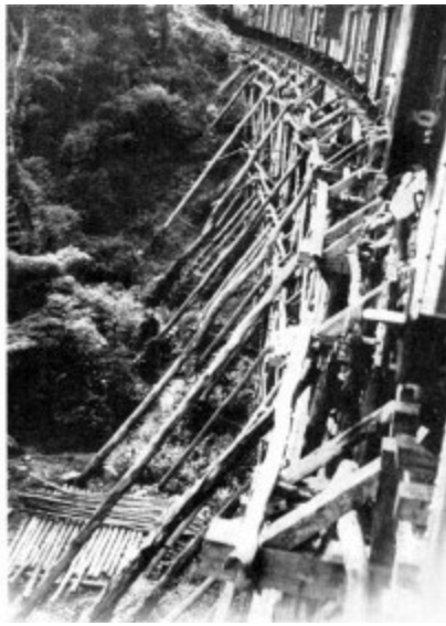
A trestle bridge on the Burma- Thailand Railway
