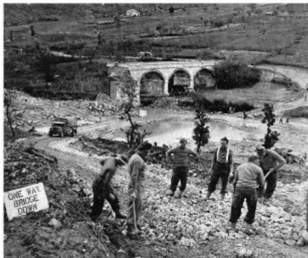
A party of New Zealand engineers repairs a deviation by a demolished bridge
