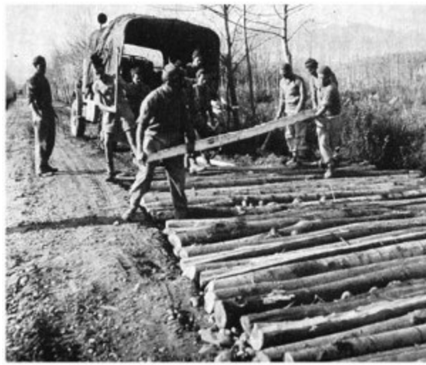
Engineers making a corduroy road up to the Sangro Engineers making a corduroy road up to the Sangro
