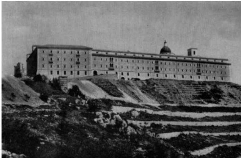
Montecassino – the south side of the rebuilt abbey
