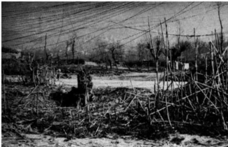
Signal wires on Route 6 Signal wires on Route 6
