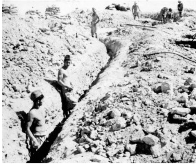
Digging a trench
